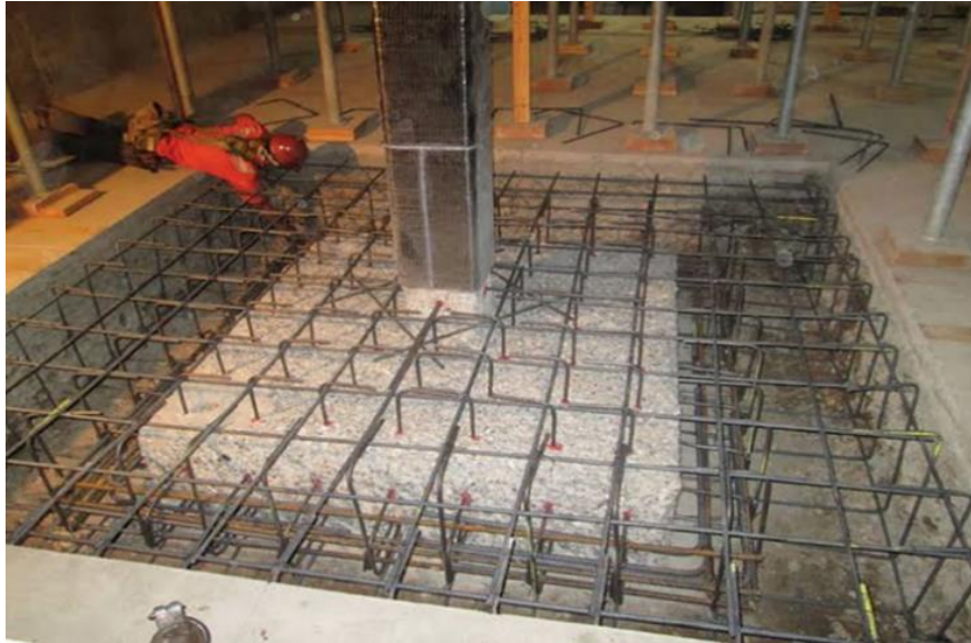
Figure 1.23 Foundation strengthening [15].
