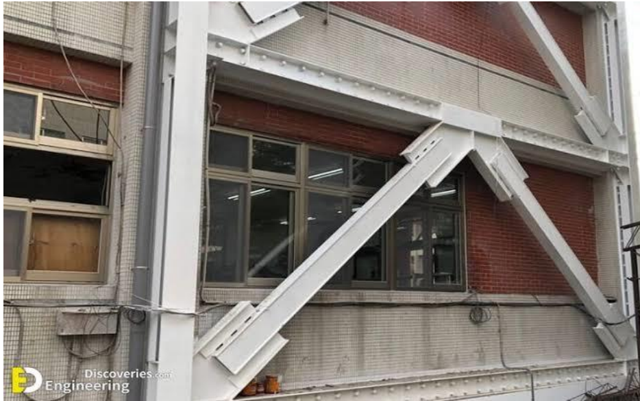
Figure 1.21 Types of bracing systems [13].
