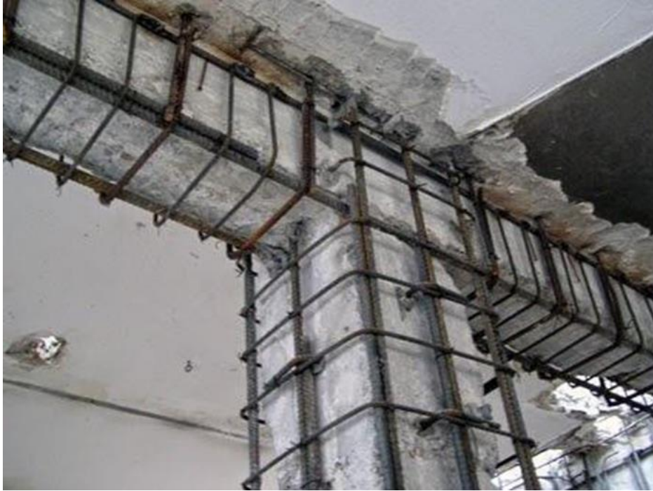
Figure 3.1. Reinforced concrete jackets [8].
