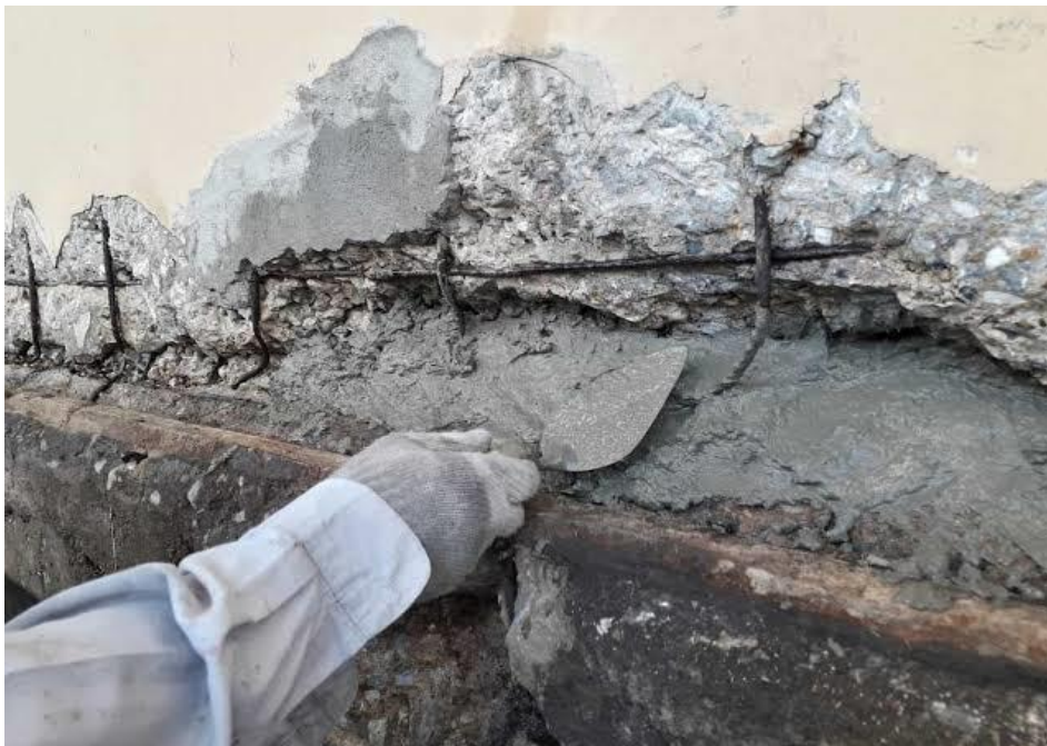
Figure 3.11. Repair with corrosion inhibitors and repair mortars [31].
