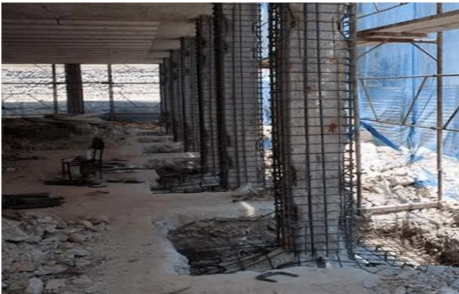
Figure 1.19 Application of RC Jackets [8].
