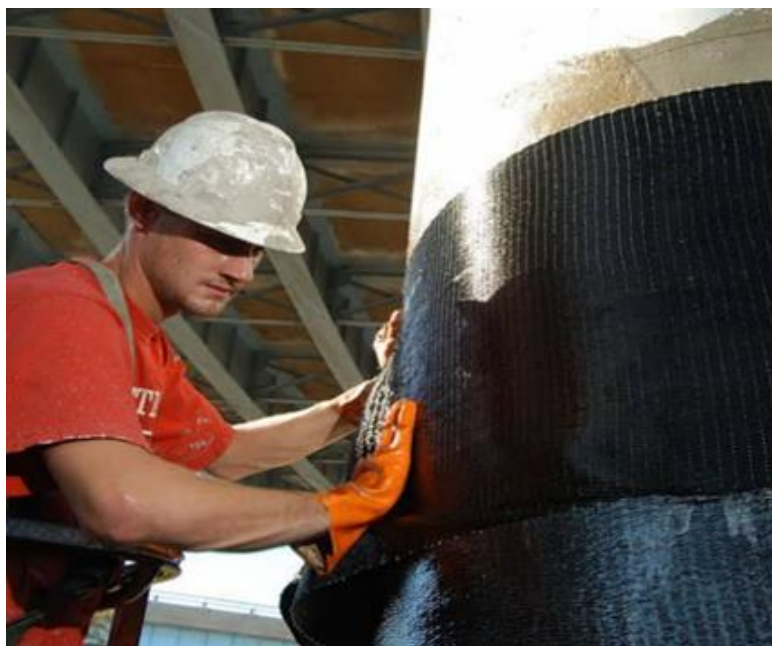
Figure 1.22 application of FRP Wrapping [14].
