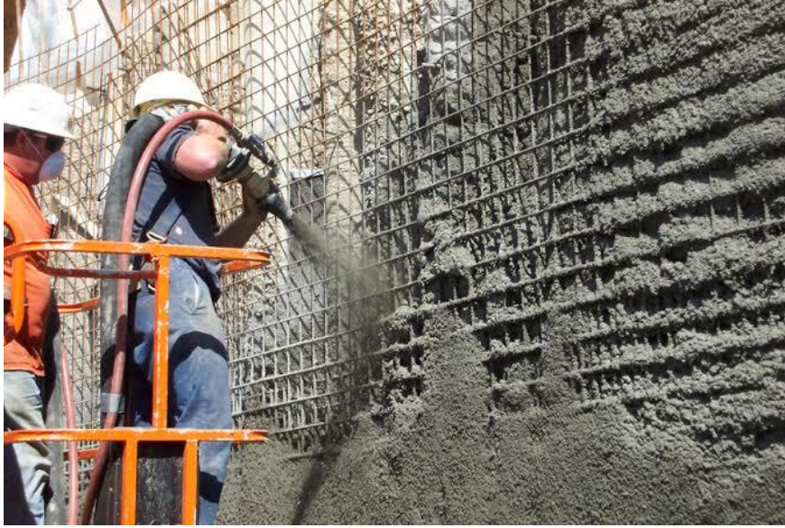
Figure 3.2 Shotcrete jacketing [27].
