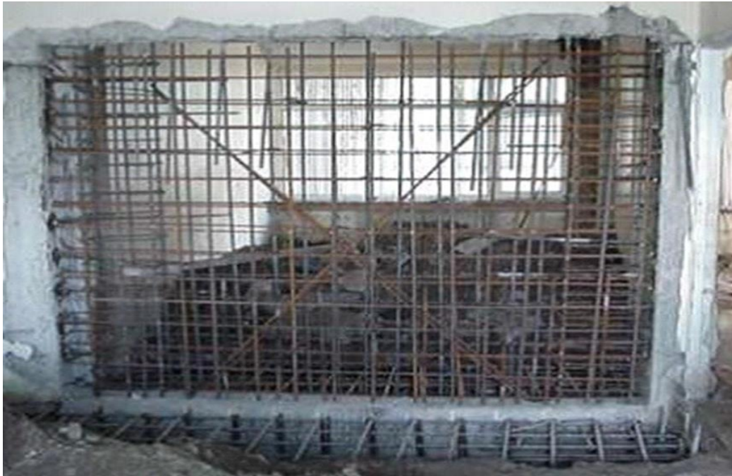
Figure 3.4 application of New shear walls [27].
