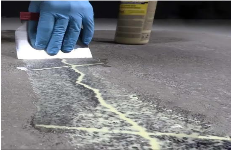
Figure 3.10. Cracks repair with epoxy resins [30].
