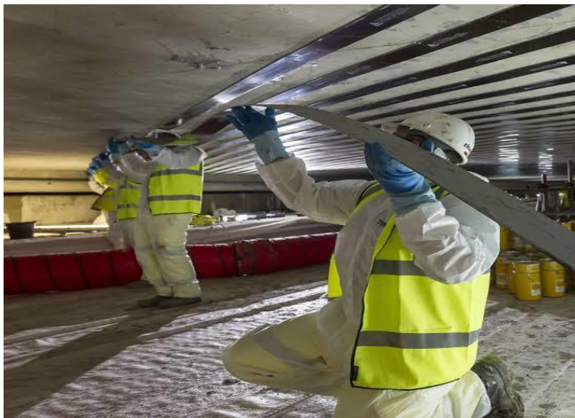
Figure 3.8 application of FRP Laminates [14].
