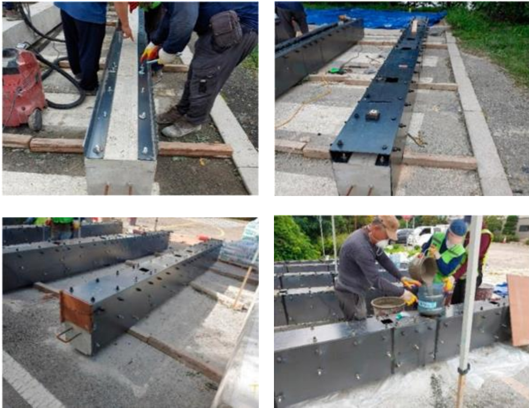
Figure 3.9 application of Steel Plates [18].
