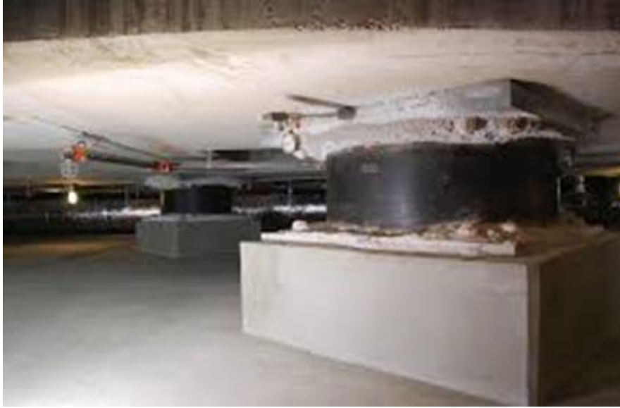
Figure 1.24 Seismic base isolation [12].
