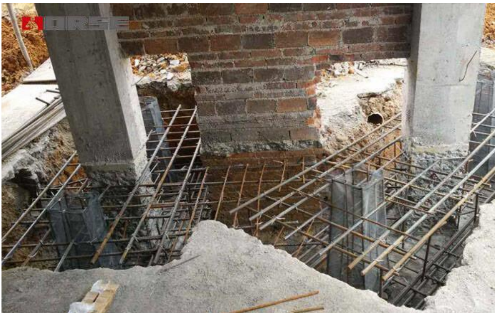
Figure 3.13. Foundation strengthening [32].
