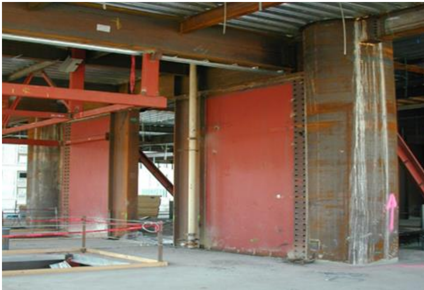
Figure 1.25 application of Steel Plates [16].
