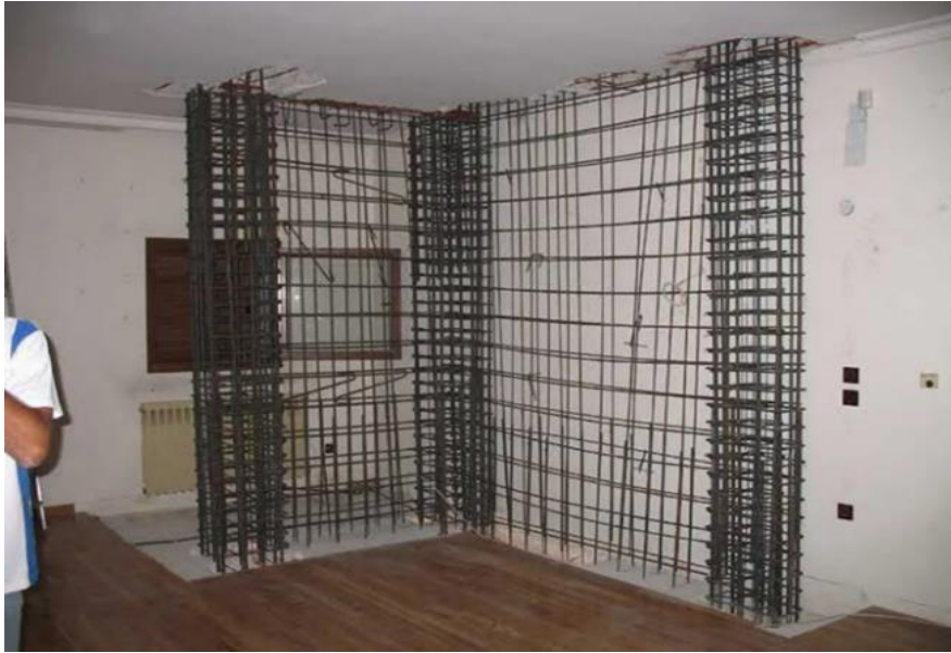
Figure 1.20 Application of New shear walls [12].
