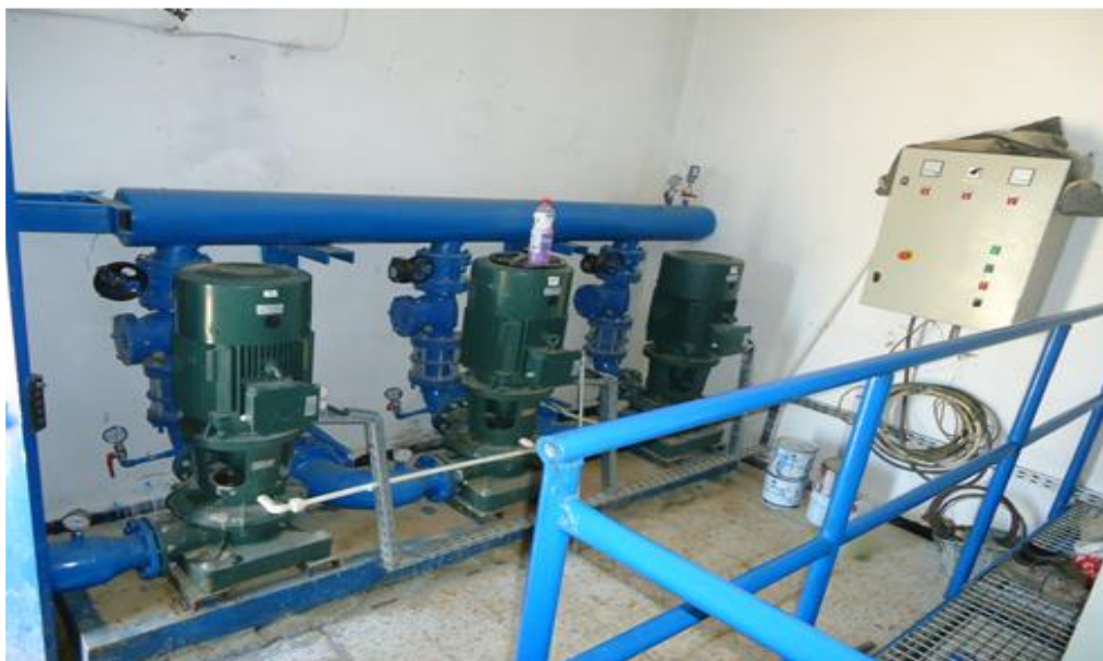
Figure VII.4: Pompe verticale
