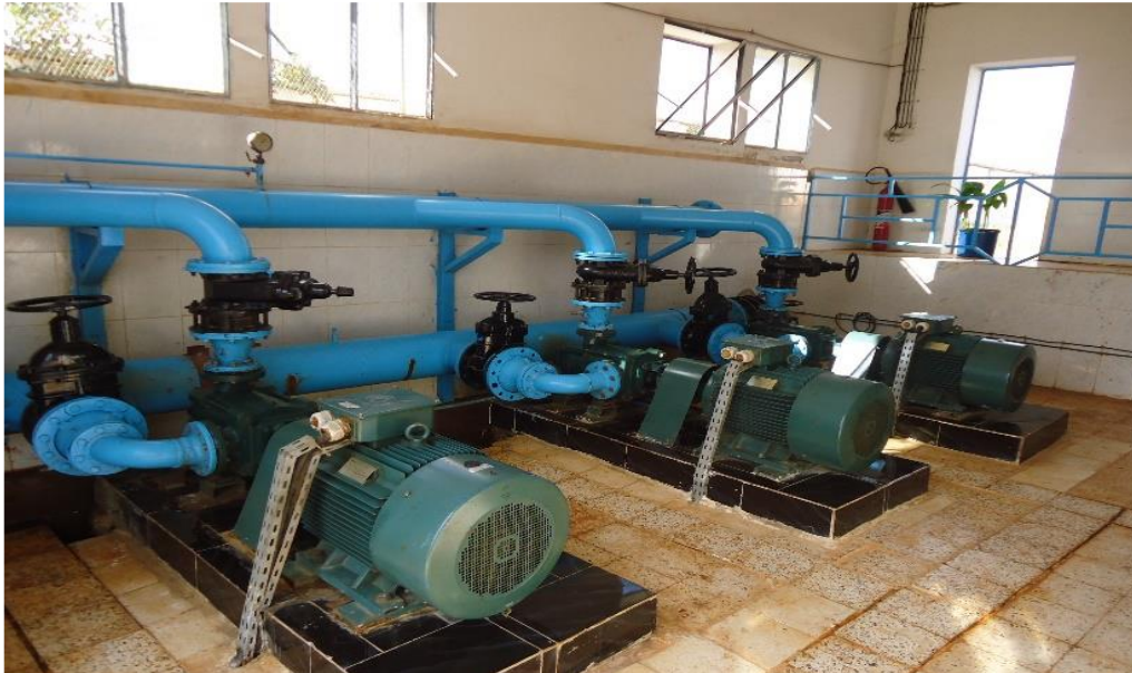
Figure VII.3: Pompe horizontale
