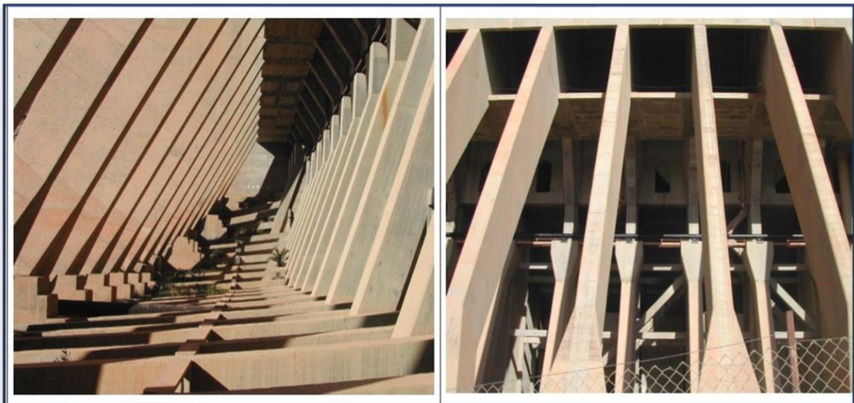
Fig.II.03. Photo des contreforts [2]
