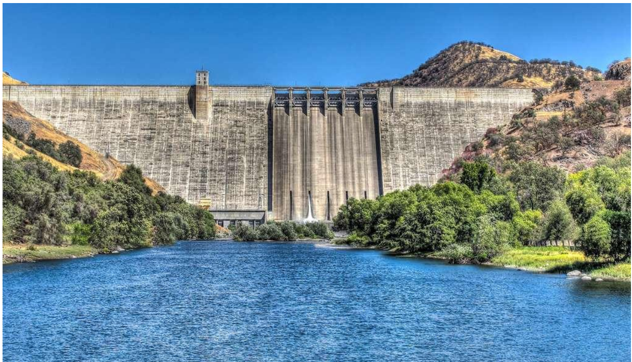
Figure I.6 : Le barrage-poids de Pine Flat
