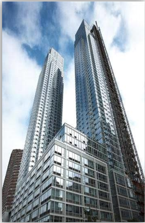
Figure .1.6 : Silver Towers Rental Building
