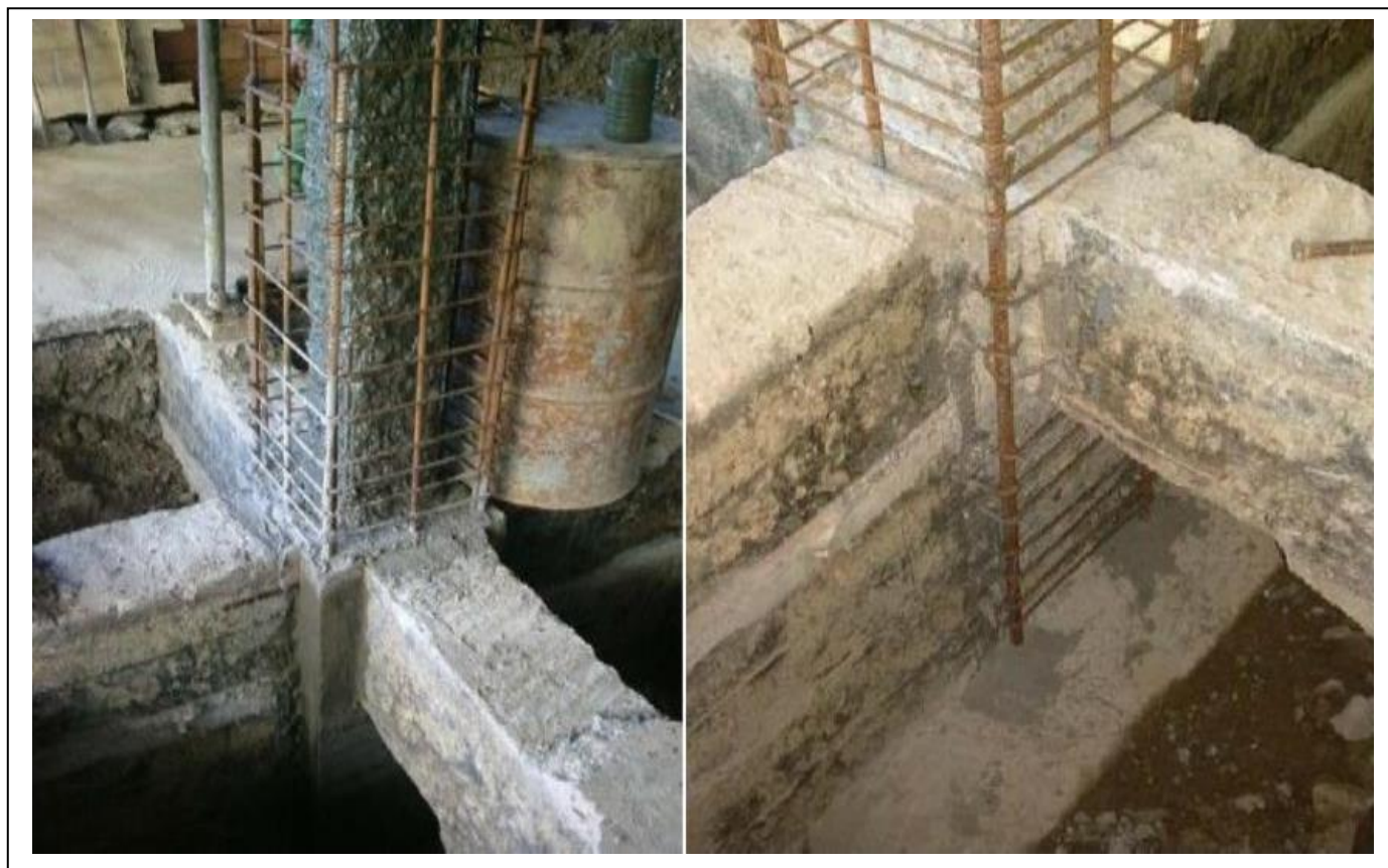
Figure III.11: Chemisage des 4 poteaux centraux
