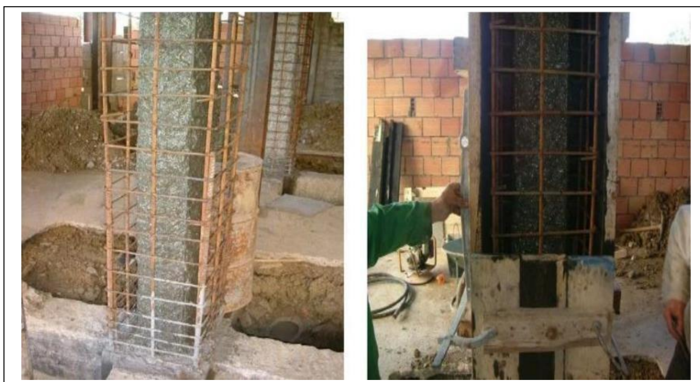
Figure III.11: Chemisage des 4 poteaux centraux
