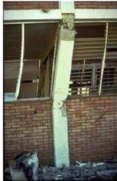
Figure II.3 : la formation des poteaux courts
