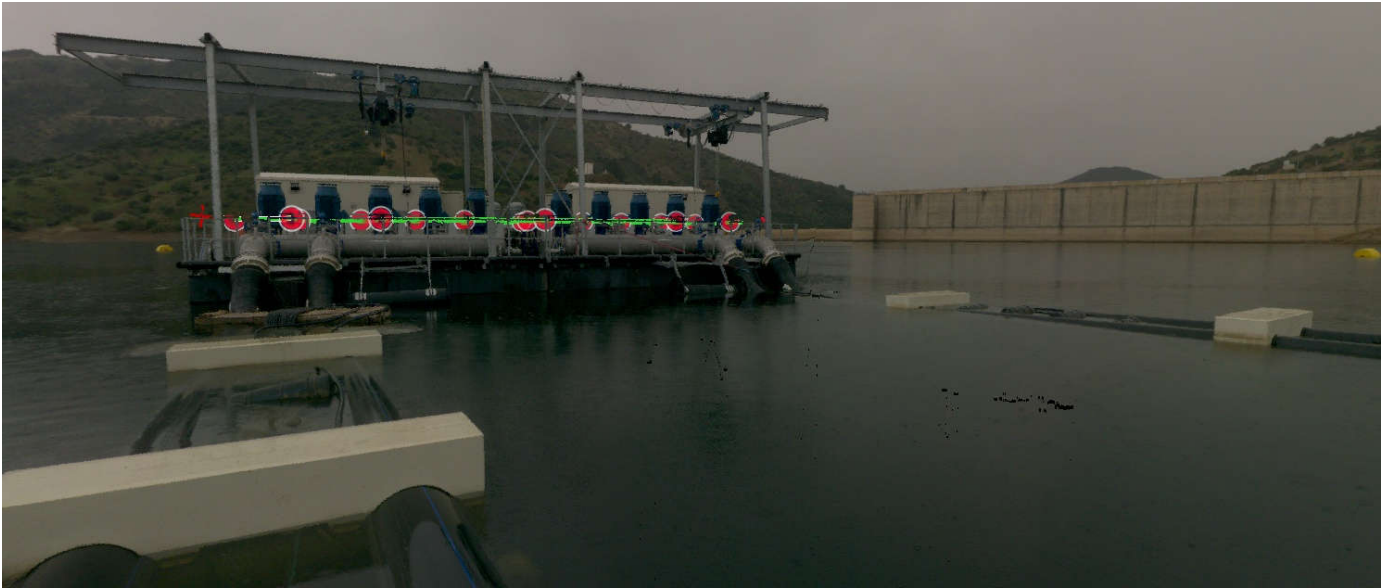
Figure 67 a 3D model of the floating pump station at oued ksob dam wall
