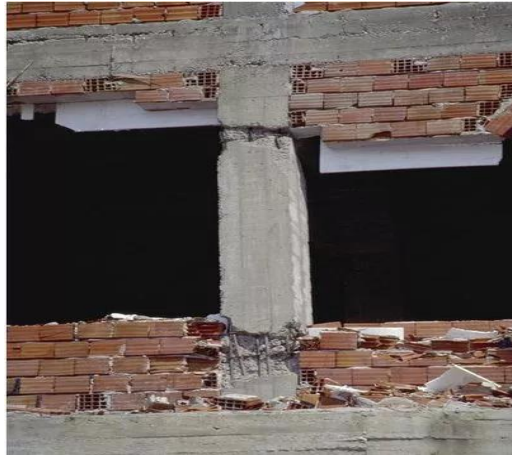
Figure II.8 : Colonne captive et colonne courte
