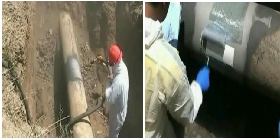
Figure IV.13 : installation de ClockSpring (STT).
