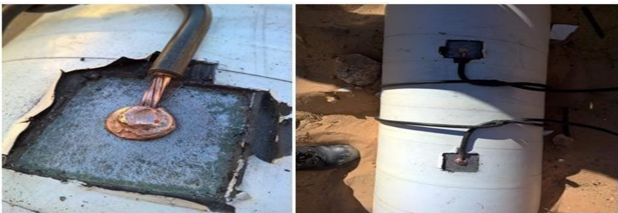
Figure II.6 Soudage des câbles de raccordement
