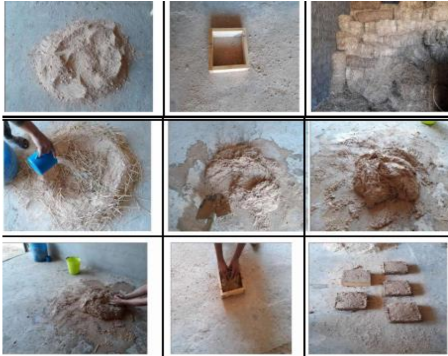
Figure II.19: Steps followed during the construction of the old brick walls.
