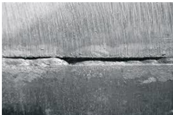
Figure I. 15 Shape of the lack of fusion defect
