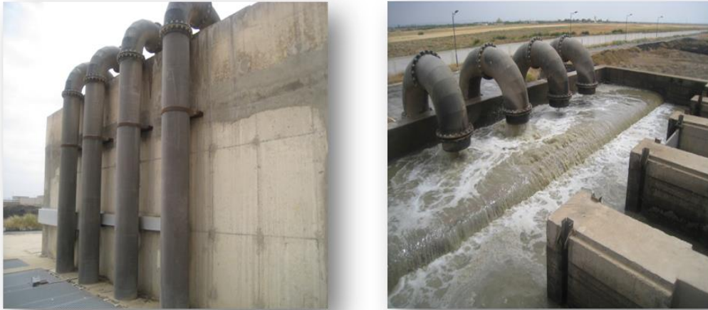
9 Fig. III. 03: La station de relevage.
