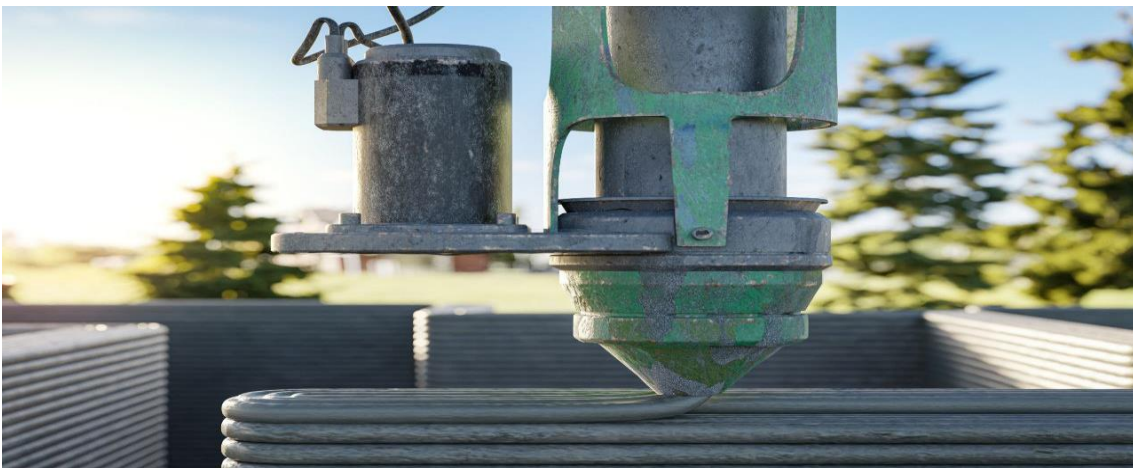
Fig. II.23. Impression 3D construction
