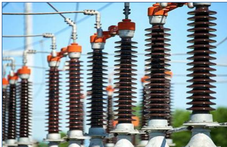
Figure 25 current transformer
