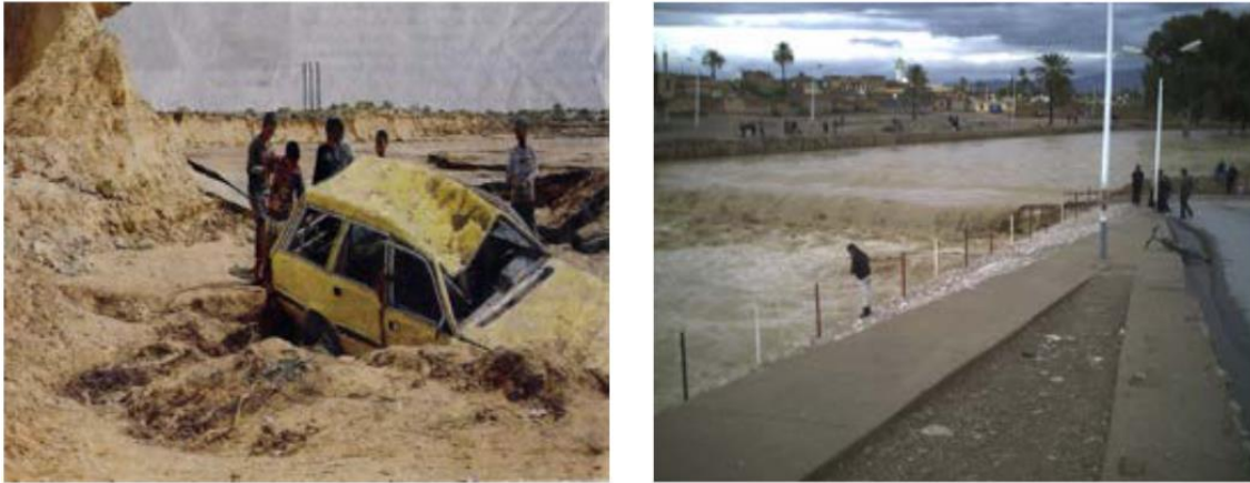
Fig. 1.9 Damages caused by floods (M'sila city, National roads 40 and 60) (Redjem et al., 2020)
