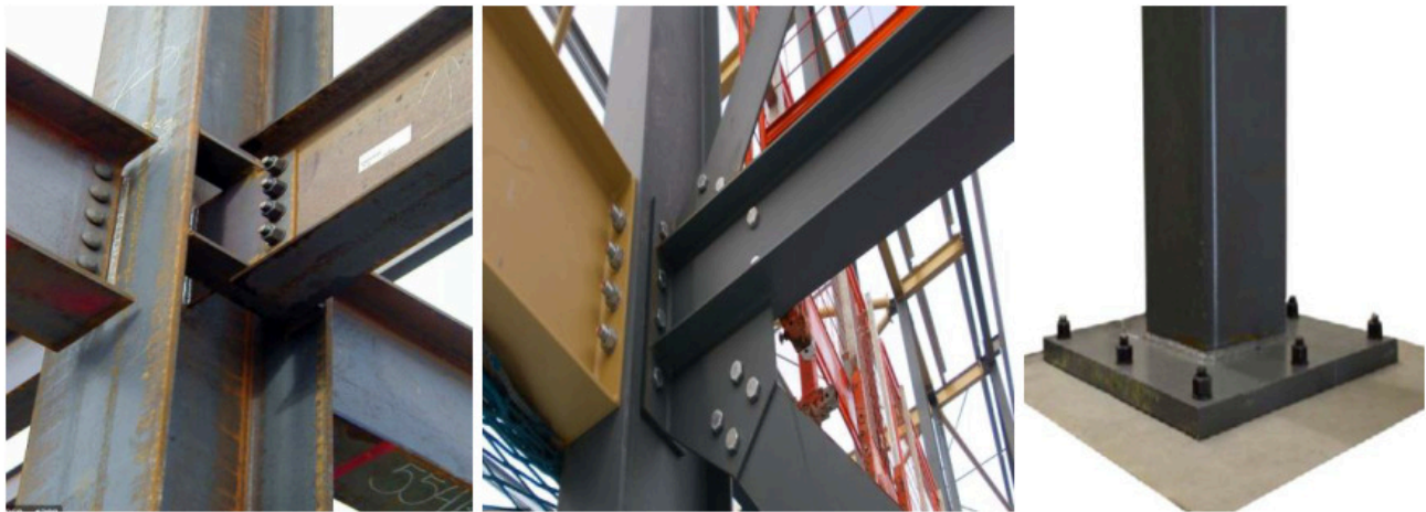
Figure 3.1. Assembly in steel structures
