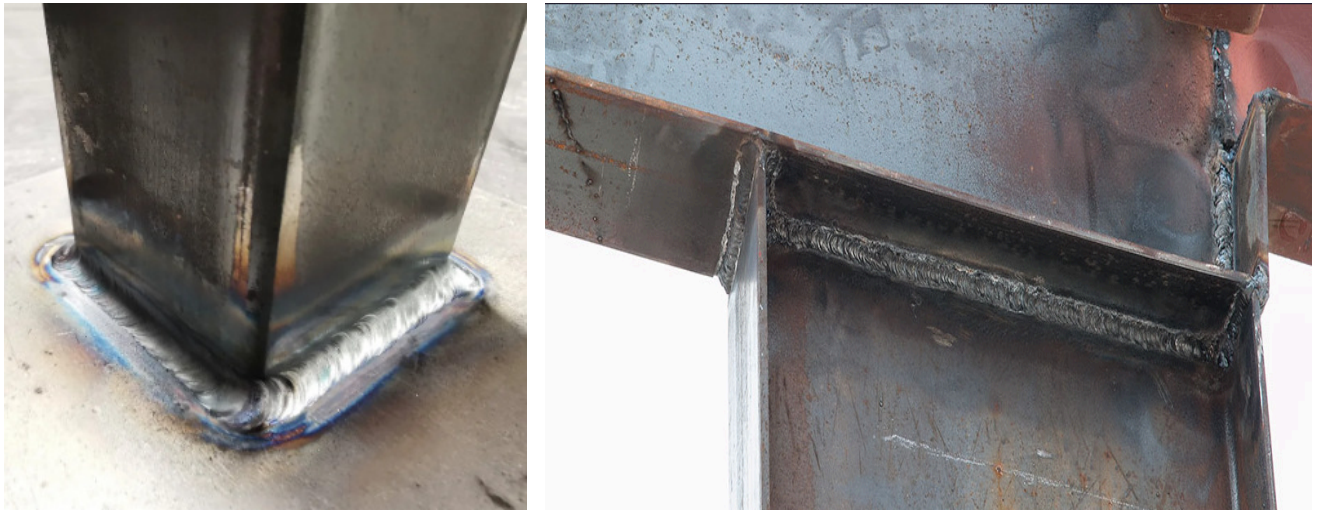
Figure 3.23. Assembly by Welding
