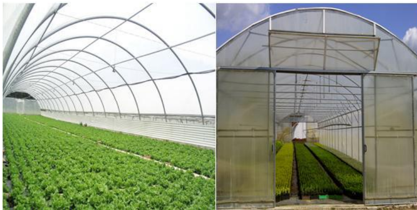
Figure 03: la serre Tunnel.
