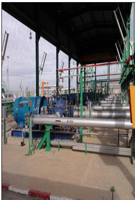
Figure (2.1) : Pompes centrifuges horizontale
