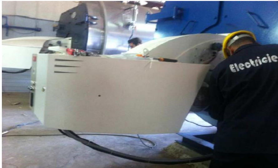
Figure IV.12. Installation of the MYRA4000 boiler at the customer's site [1].
