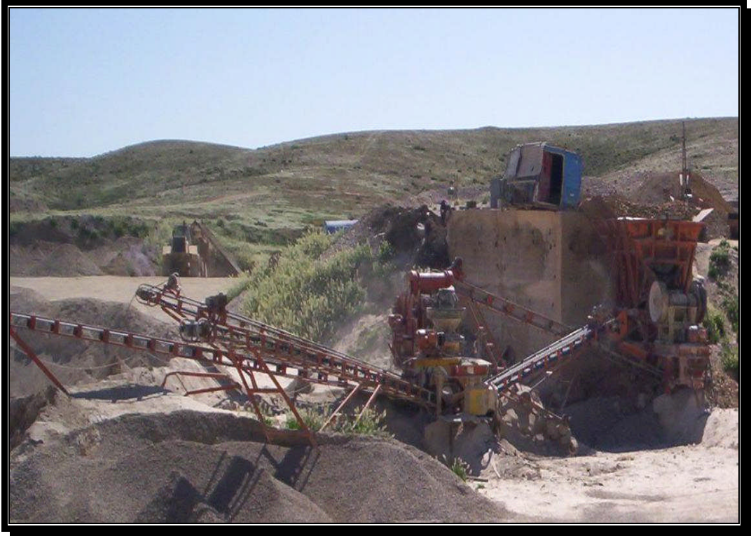
Fig. I.3: Station de Concassage 100t/h.
