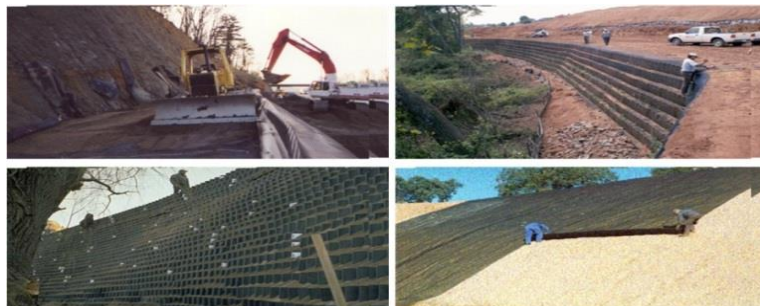
Figure I.25: Application géotextiles.
