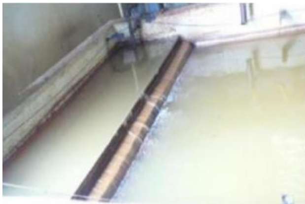
Figure IV-3: Corrugated Plate Interceptor CPI « S-102 »
