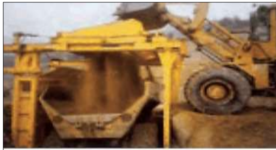
Figure V.34 : Criblage (source SETRA).
