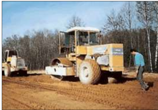
Figure V.40 : Compactage (source : SETRA).
