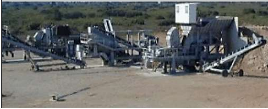
Figure V.35 : Criblage (source SETRA).
