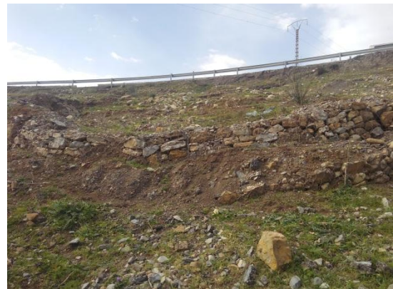
Figure II.3 : Gabion endommagé
