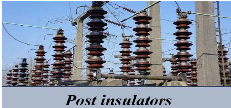
Figure I.9. Post insulators.
