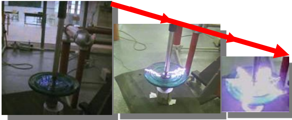
Figure I.13. Flashover high-voltage insulators.
