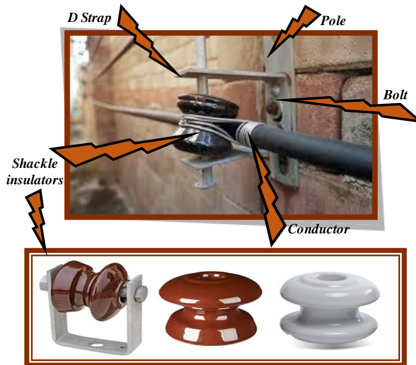
Figure I.6. Shackle insulators.
