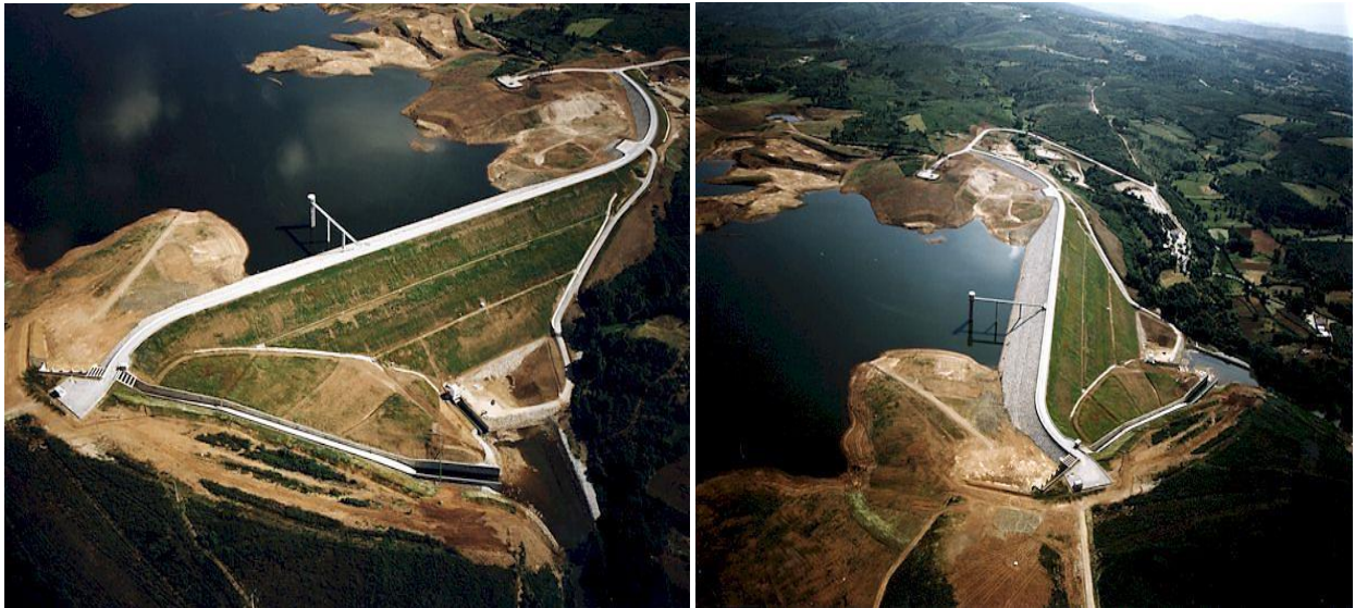
Figure I-3: Barrages en terre (Sabugal)
